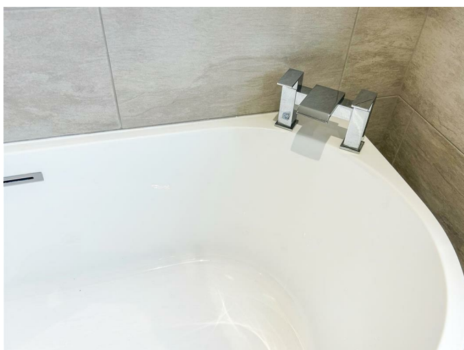
The Bathroom Finishes
